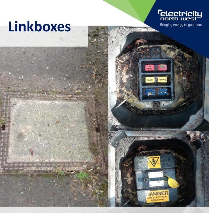
Linkboxes can be found in underground sections of our network often in the pavements. They are recognisable by their covers and they are used to connect multiple sections of underground cables together. If you ever have a power cut, you may see our engineers using these boxes to isolate the fault or to restore the supply.
