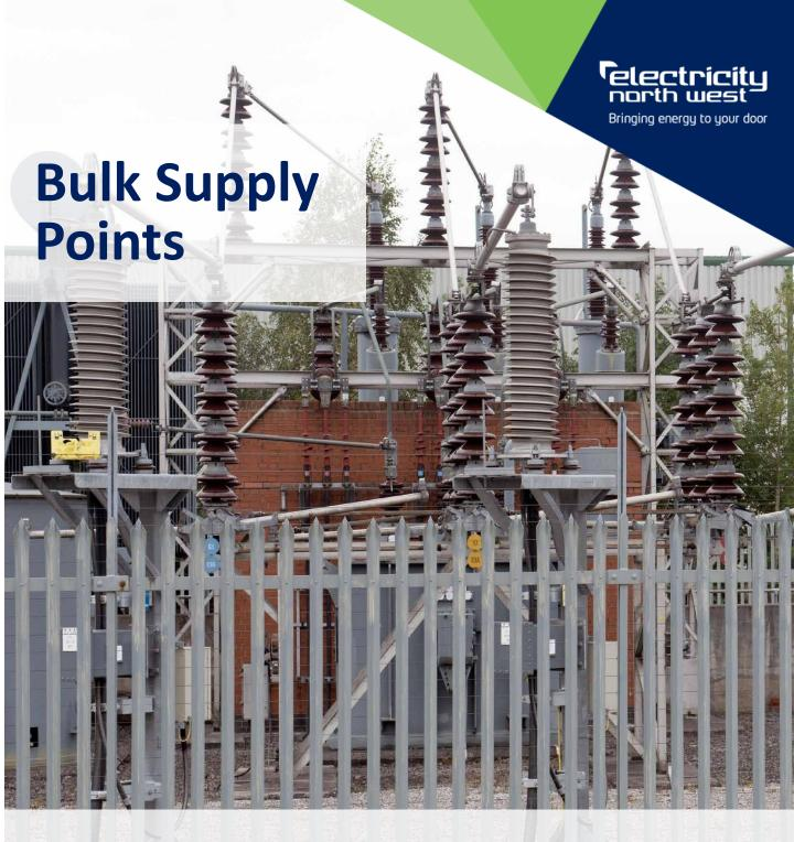
Bulk Supply points are sections on our network which connects the transmission section of our network to the distribution section of our network. Power comes in at 132kV and is transformed down to 33kV, before being distributed to our primary substations.
