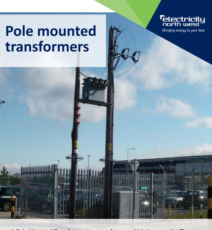
A Pole Mounted Transformer is a transformer which is on a pole. They are the same as a transformer on the ground, just on a pole. These are usually found on our overhead sections of our network but can be used when there isn't enough space on the ground for a regular substation.
