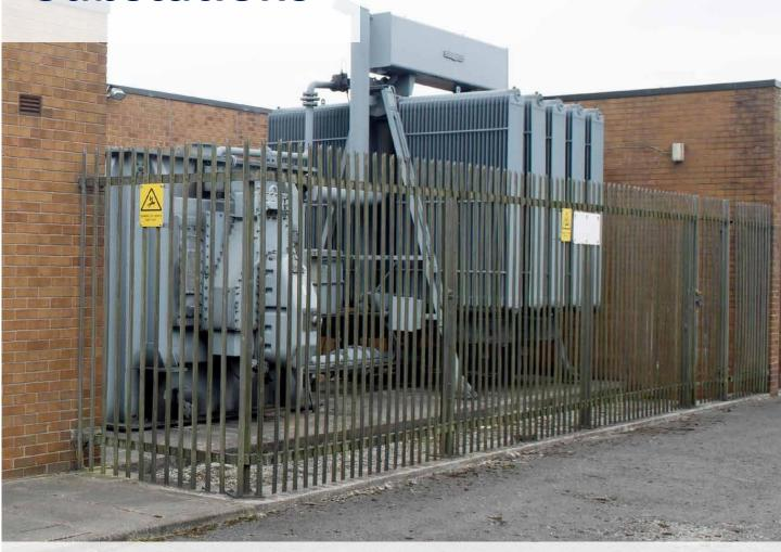
Primary substation are points in our power system where power is transformed from 33kV to 11kV or 6.6kV. These can be found all around our network and can be inside buildings or outside. The use of extra high voltage allows us to distribute electricity in large quantities and safely.
