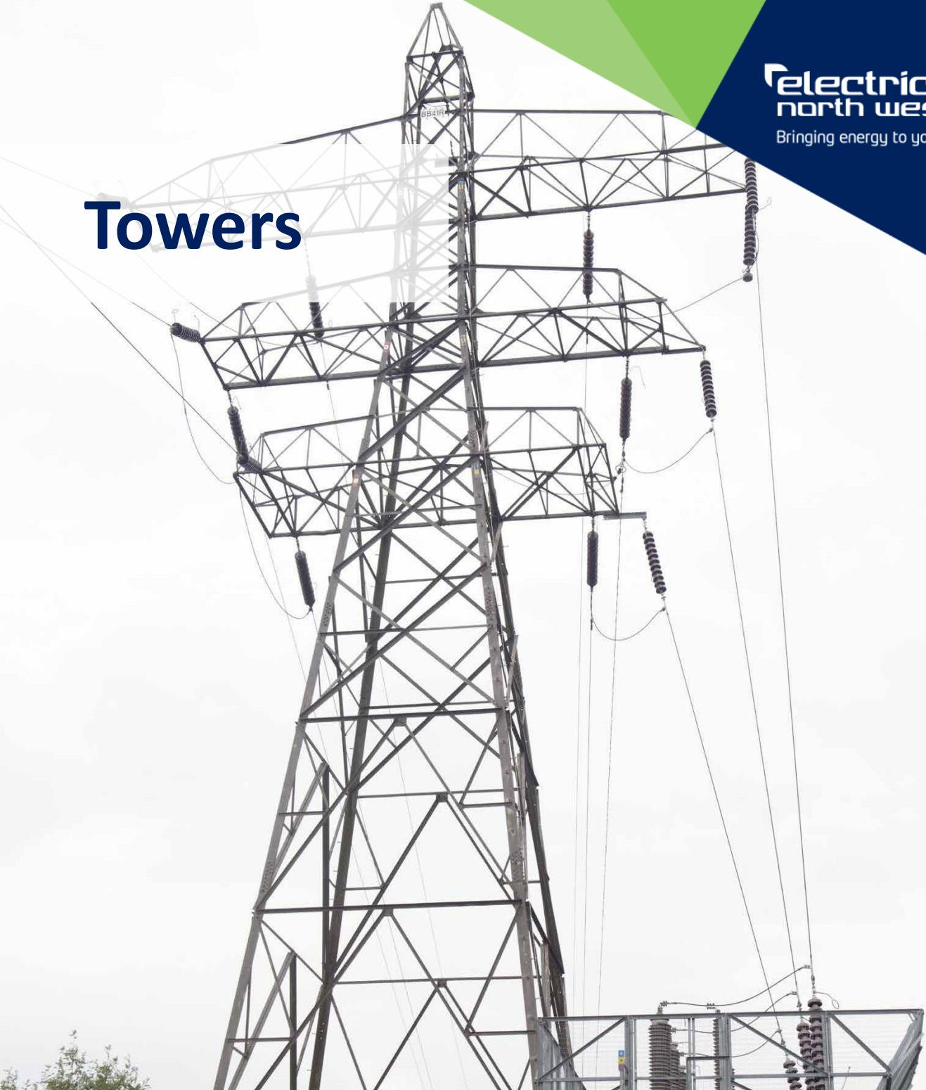
Towers are used to carry extremely high voltage transmission lines that transport bulk electricity from generating stations to electrical substations. We use them to transmit electricity at 132kV from our Grid Supply Points to our Bulk Supply Points and our Primary substations.
