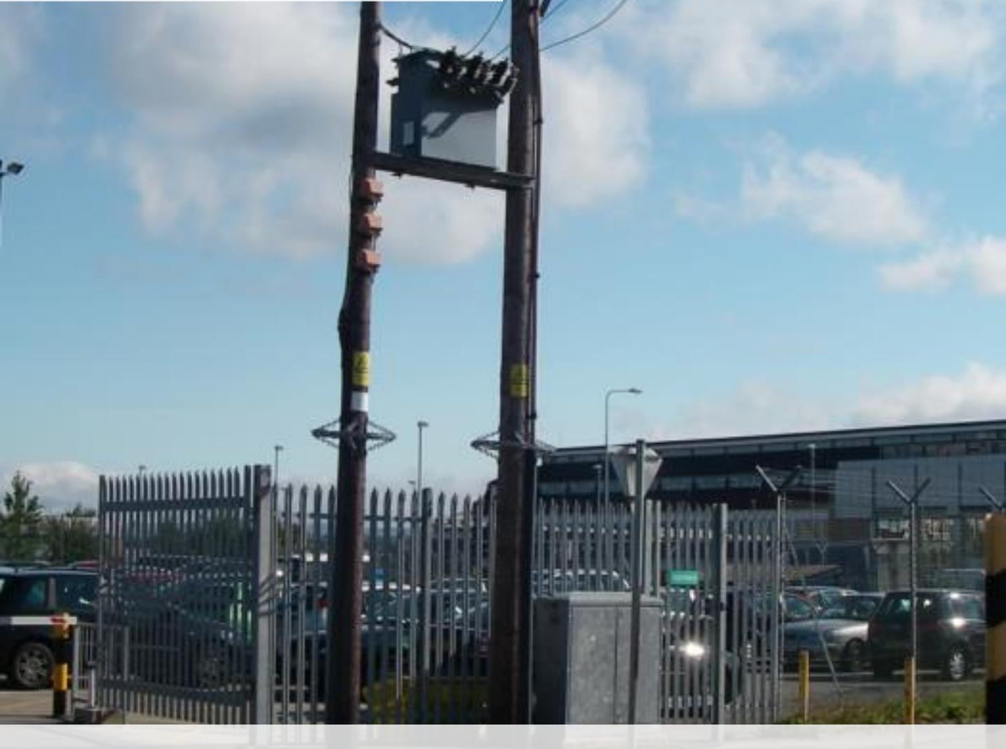
A Pole Mounted Transformer is a transformer which is on a pole. They are the same as a transformer on the ground, just on a pole. These are usually found on our overhead sections of our network but can be used when there isn't enough space on the ground for a regular substation.
