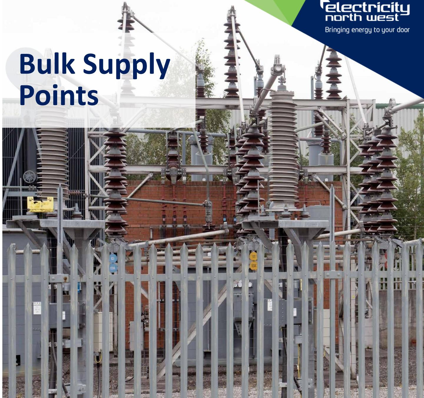
Bulk Supply points are sections on our network which connects the transmission section of our network to the distribution section of our network. Power comes in at 132kV and is transformed down to 33kV, before being distributed to our primary substations.
