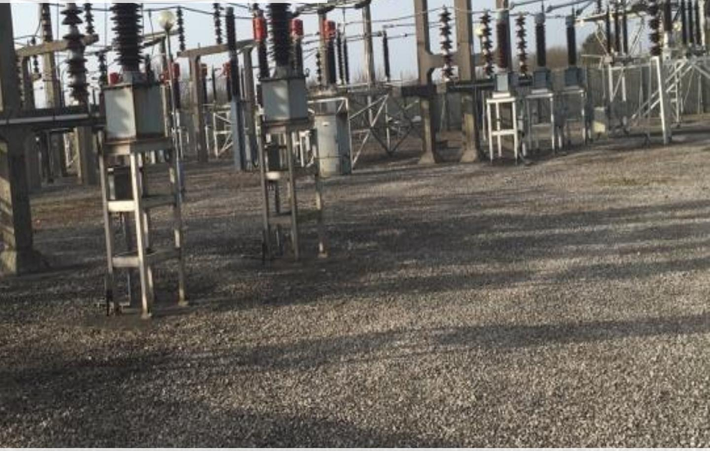
Grid Supply Points or GSP for short is the section of the electricity network where we take over from National Grid. These substations are located at 18 key areas across the North West. These can be spotted as very large substations as electricity cables come in at 400kV or 275kV and using transformers we bring this down to 132kV or 33kV to transmit across the North West safely.
