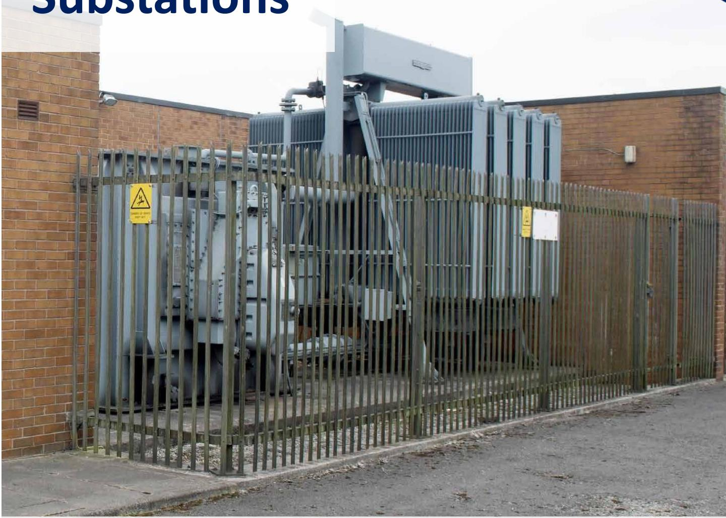
Primary substations are points in our power system where power is transformed from 33kV to 11kV or 6.6kV. These can be found all around our network and can be inside buildings or outside. The use of extra high voltage allows us to distribute electricity in large quantities and safely.
