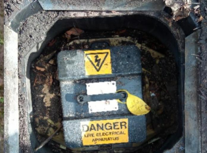
Linkboxes can be found in underground sections of our network often in the pavements. They are recognisable by their covers and they are used to connect multiple sections of underground cables together. If you ever have a power cut, you may see our engineers using these boxes to isolate the fault or to restore the supply.
