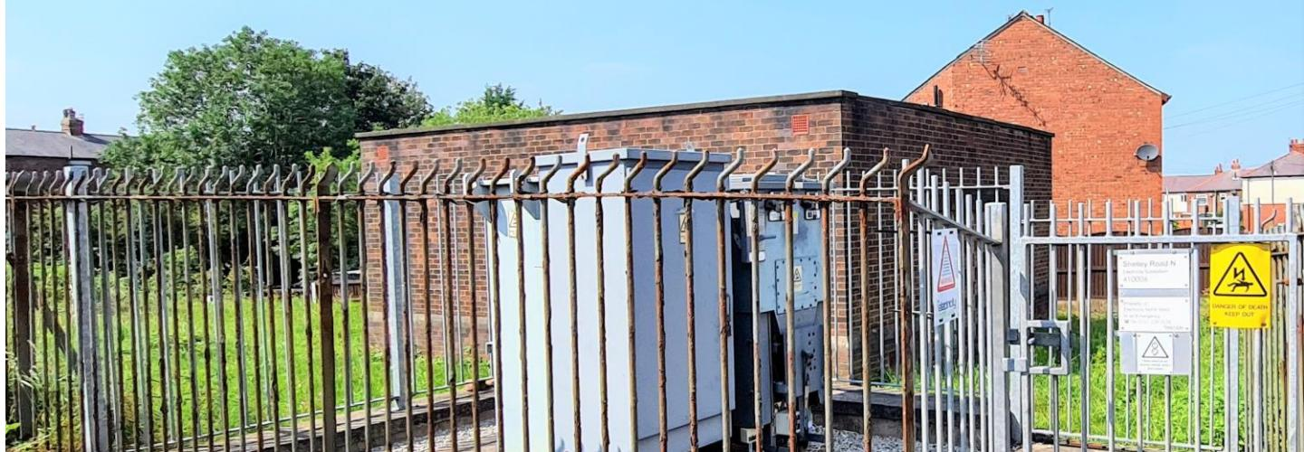
Distribution Substations are points on our network where electricity is transformed from high voltage (11kV or 6.6kV) to low voltage (400V) to allow electricity to be passed through cable to your homes. These will typically be found nearby to houses and sometimes in between houses. They can be situated in a building or a fenced area depending on the location.
