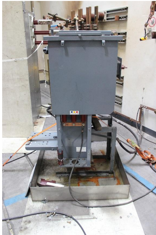
Photo No. 08: After test XZ 289 F 005 / 011 Test object, side view
