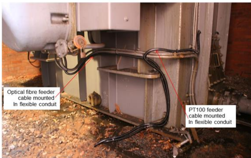
Figure 4-3 Routing of the optical fibre feeder and PT100 flexible trunking
