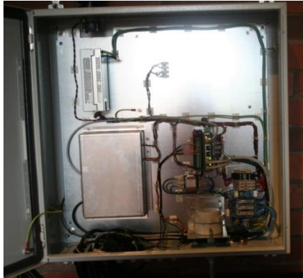
Figure 4-5 Communications enclosure (external and internal views)
