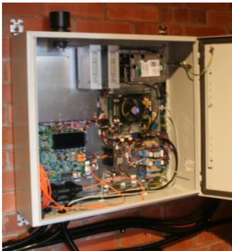
Figure 4-6 Acoustic enclosure (external and internal views)
