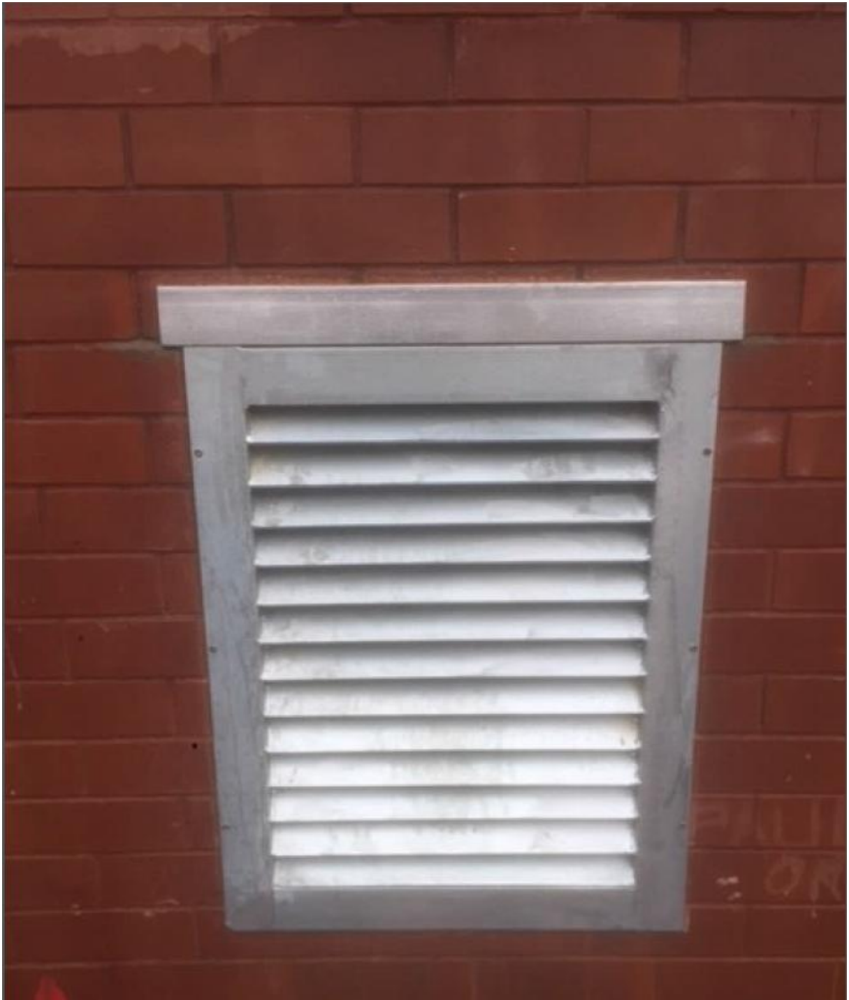
Figure 3: Additional vent on a brick built substation (external)
