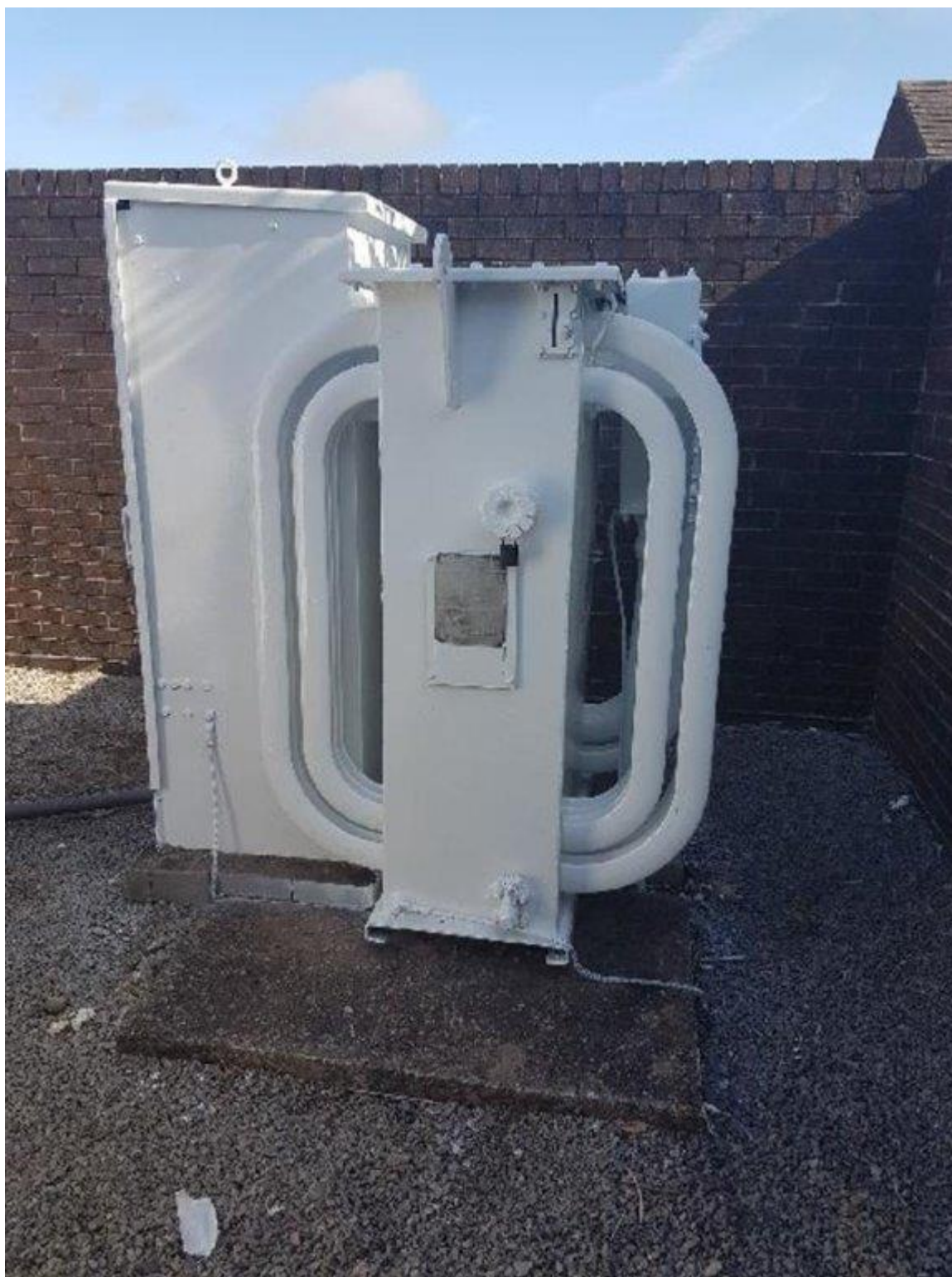
Figure 6: Transformer painted with solar reflective paint
