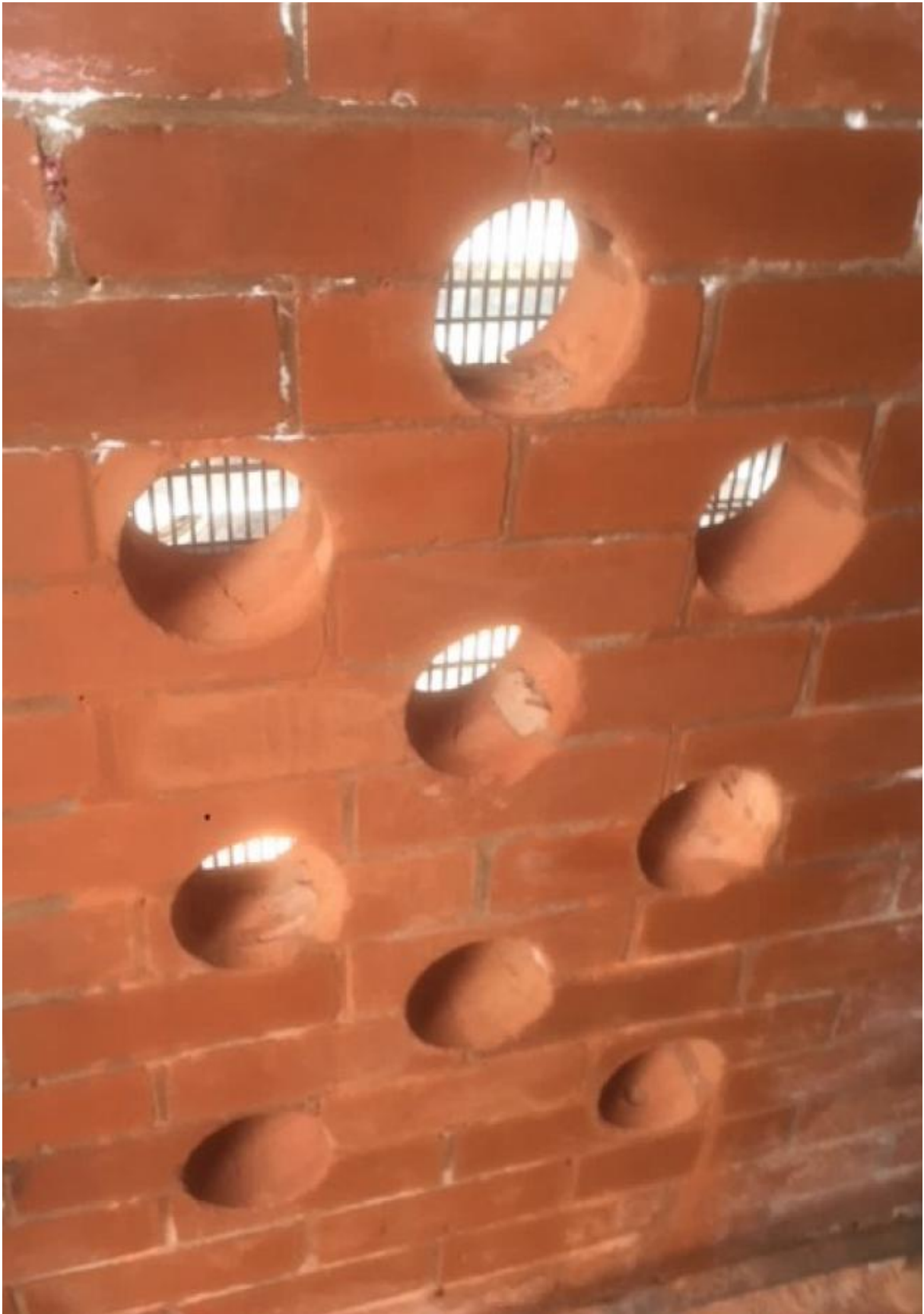
Figure 4: Core drilling on internal substation wall
