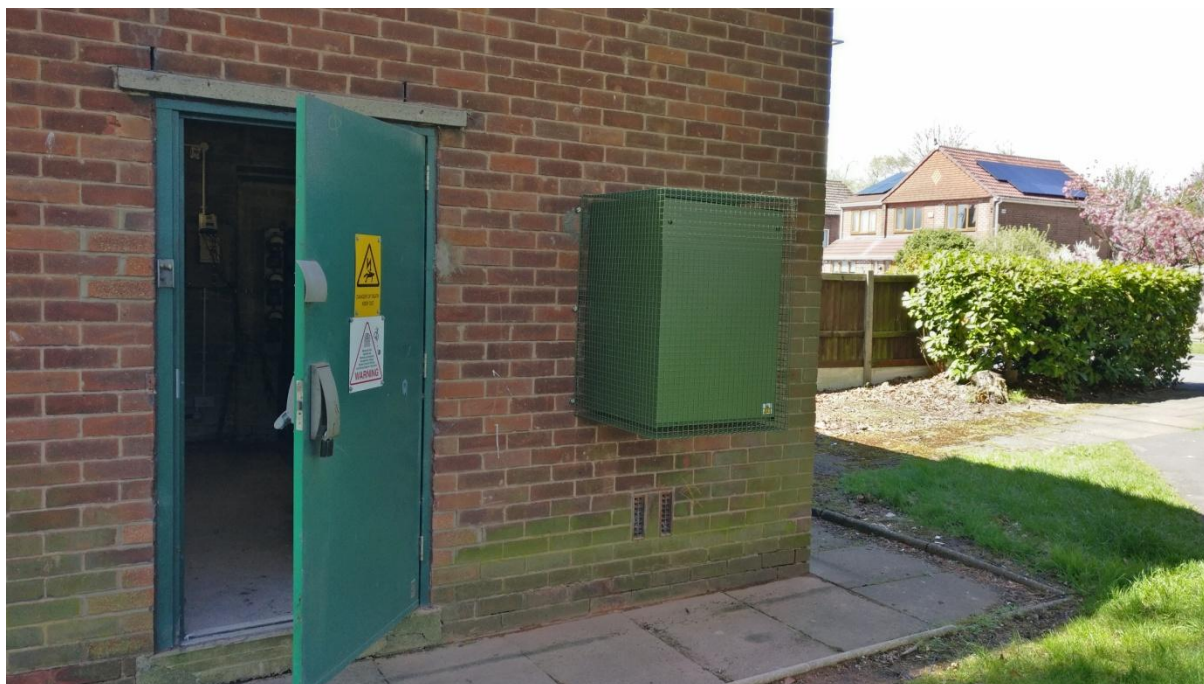
Figure 2: Externally mounted Passcomm install
