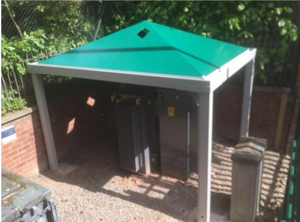
Figure 7: Transformer covered with shading canopy
