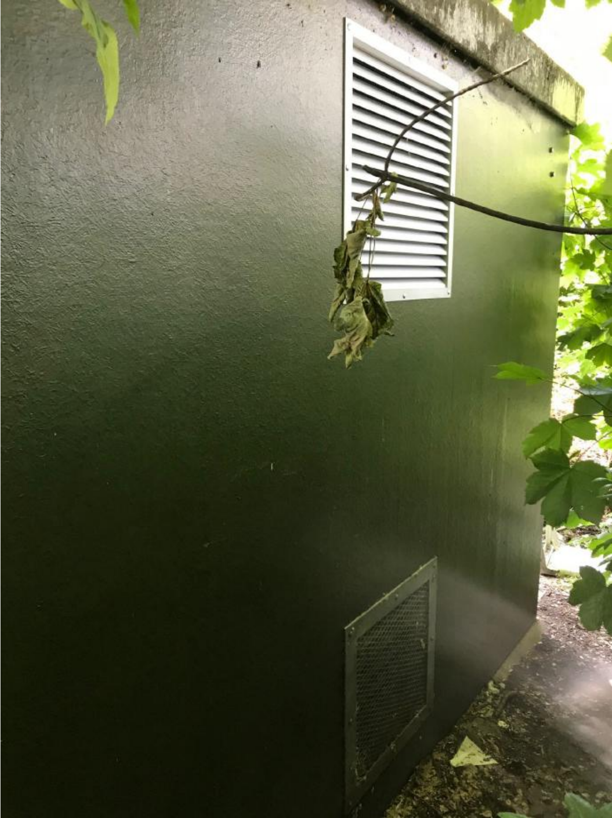
Figure 5: Additional vent fitted to a GRP substation
