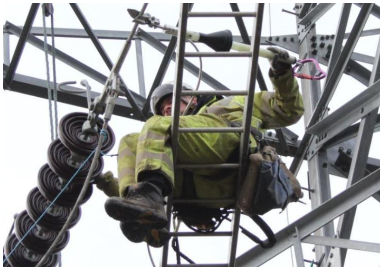
Bridging earth for insulators (with angle type conductor clamp) (also used with normal type conductor clamp)
