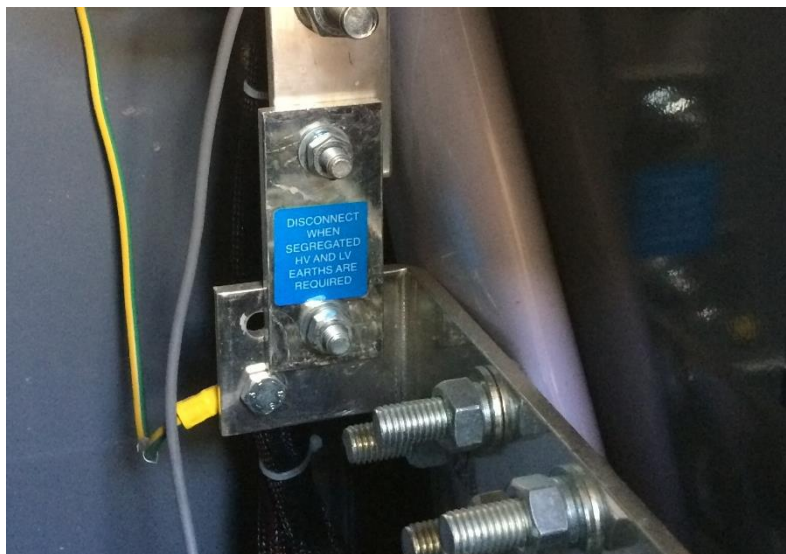
Fig. 4 – Typical HV – LV Earth Link (Combined HV and LV Earthing Systems Shown as Link is Present)
