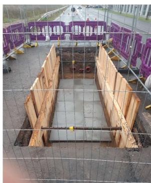
If a canopy is specified, this shall be constructed to provide adequate protection for operatives working in the joint bay and be capable of withstanding wind loads and other climatic conditions typically expected in the North West of England. The canopy shall have a waterproof sheet securely tied to a suitable tubular frame scaffold fixed rigidly to the joint bay sides.
