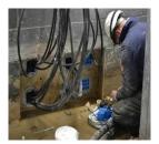
Roxtec UG™ Sealing Solution; A visual inspection of the Roxtec sealing system after installation is sufficient.
