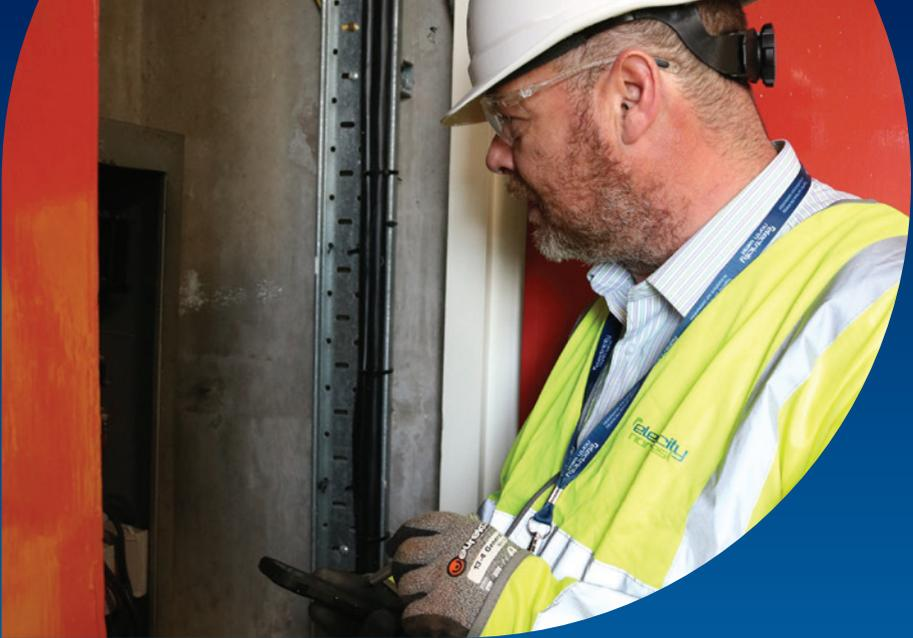
Rising and Lateral Mains (RLM) is the name we give to the electrical distribution system in multi-occupancy buildings such as flats. Electricity rises through the building on mains cables and laterally through service cables to individual properties to provide them with power. We're responsible for providing you with a safe supply of electricity up to our cut-out, a piece of equipment that connects your electricity meter to our system.
