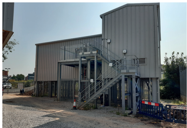
Rochdale Central - 6.6kV Elevated switchroom
