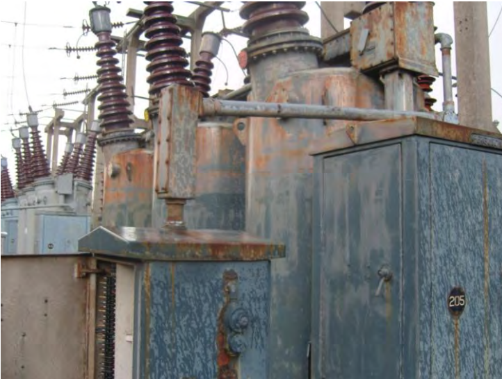
Corroded circuit breaker tank at Padiham
