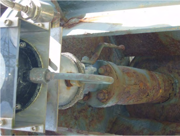
SF 6 Receiver showing corrosion at Peel
