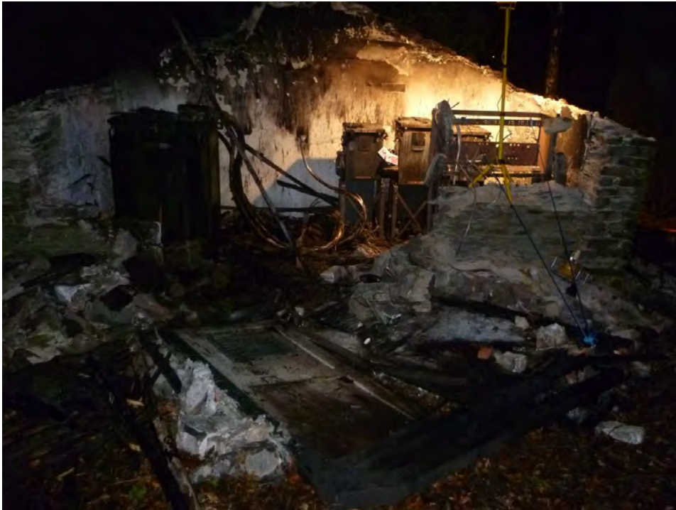
Aftermath of disruptive failure of GF3 fuse switch at Scale Howe s/stn, Ambleside.
