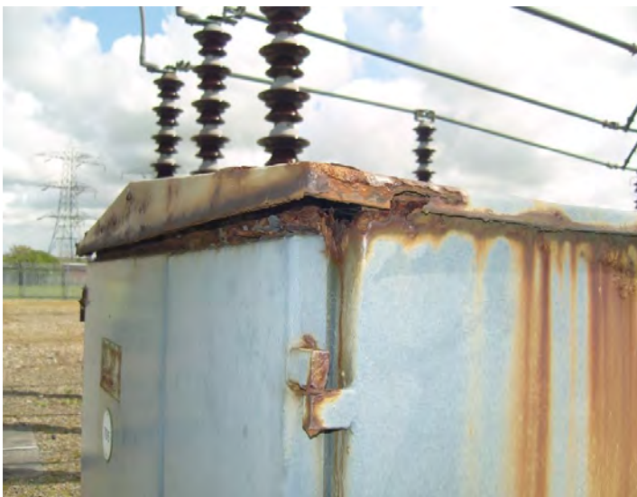
Heavily corroded marshalling kiosk at Peel
