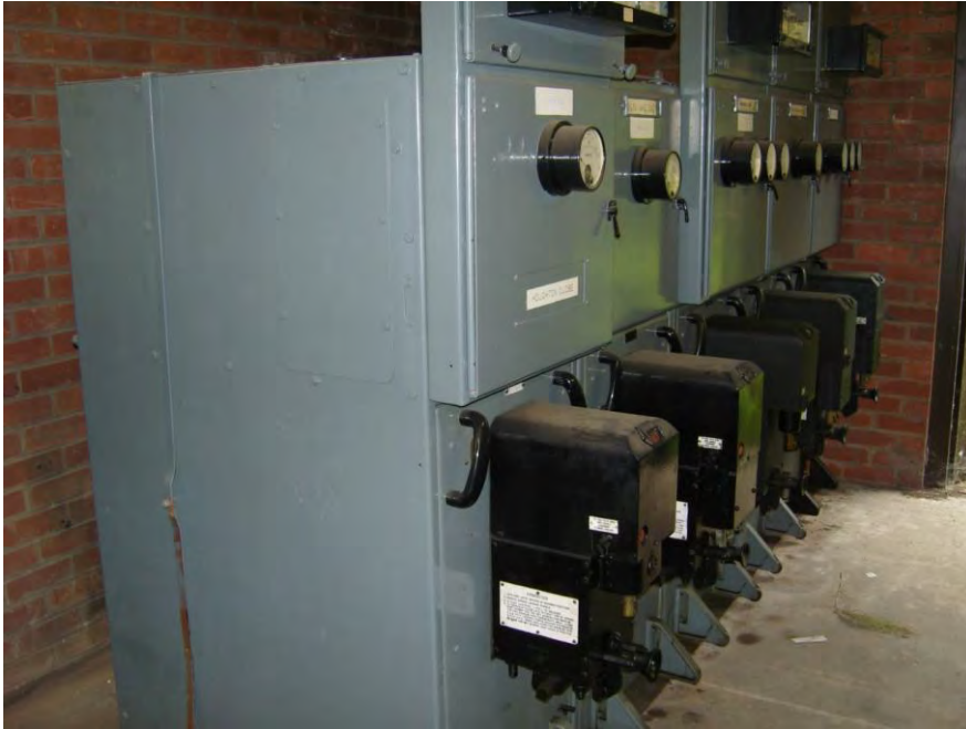
HV switchgear panel requiring extensible switchgear replacement solution
