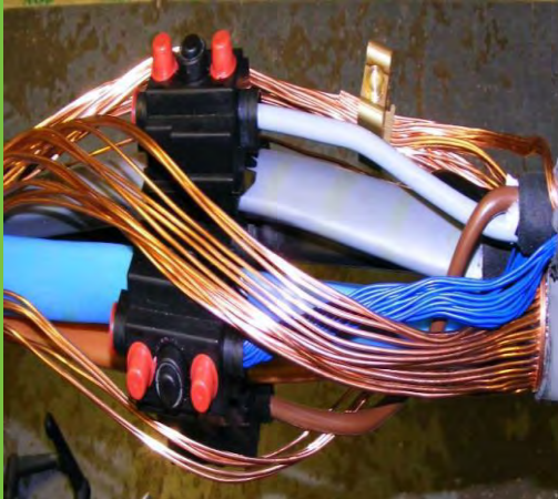
Low voltage smart joint
