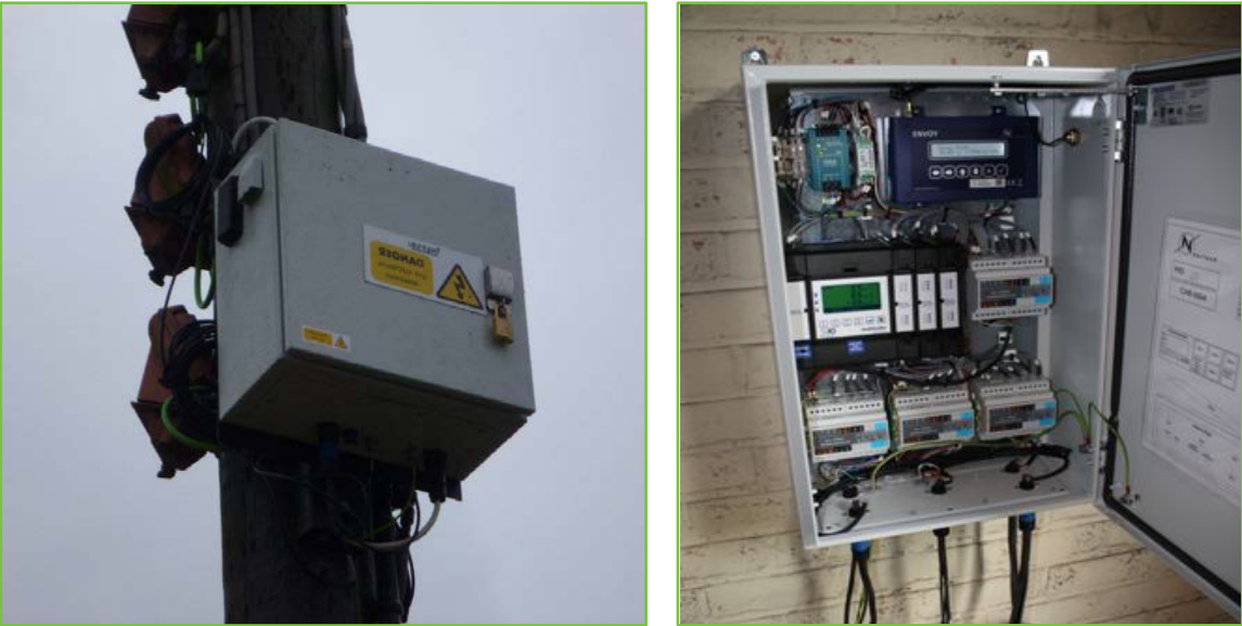
Figure 3 – Nortech substation monitoring on a pole (left) and indoors (right)
