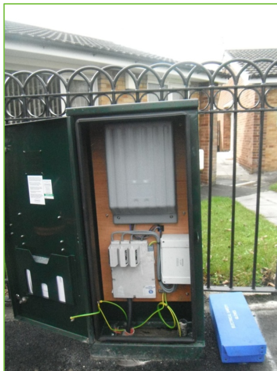
Figure 5 – Housing containing GridKey data concentrator
