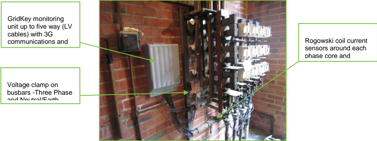
Figure 3 – Nortech substation monitoring on a pole (left) and indoors (right)
